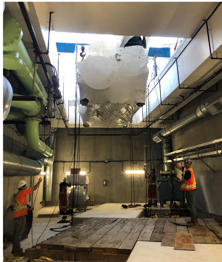
Delivery to the False Creek Energy Centre
